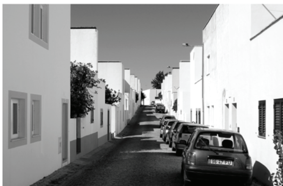
Aspect of street in the area developed for the members of the Giraldo Sem Pavor Cooperative (top) and Boa Vontade Cooperative (bottom). Situation in 2011. Photos: Nelson Mota.
